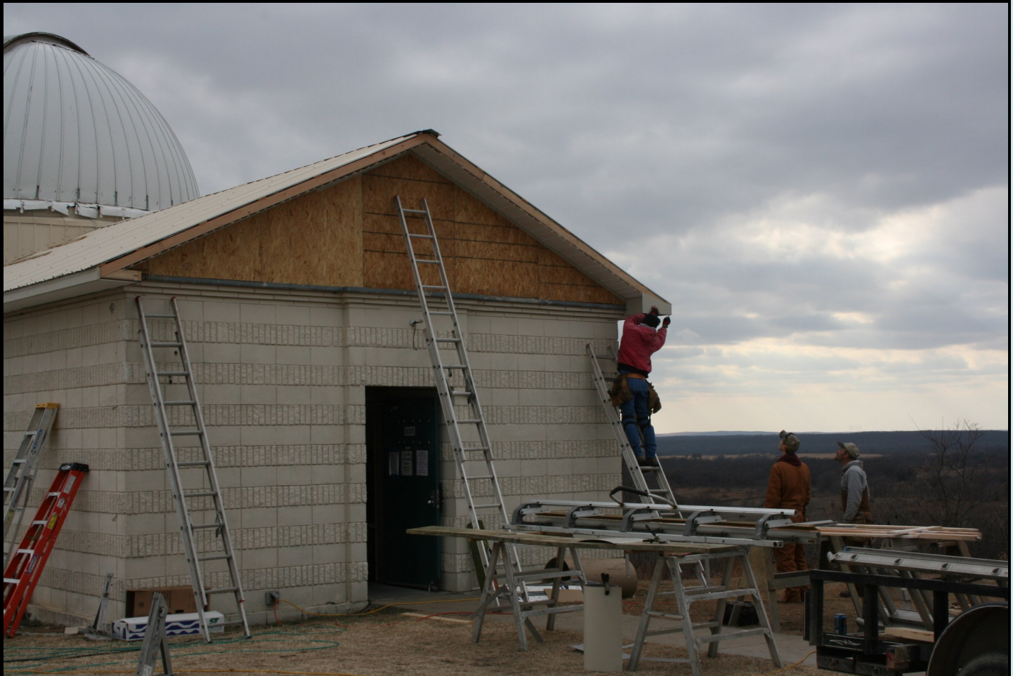
Photo: Work in Progress at the Observatory, January 2014, by Tamara Green.
